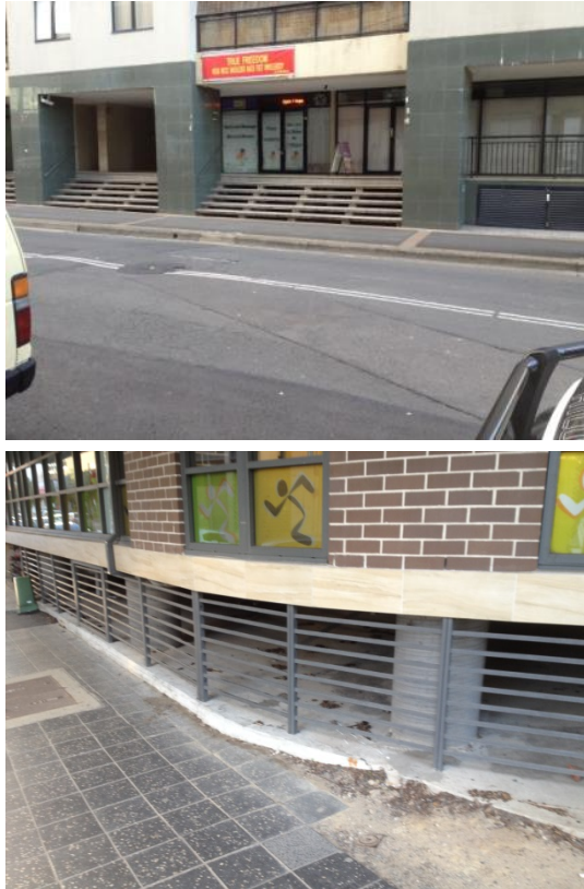
Figure 12. Examples of ground floor levels raised to meet minimum floor level and flood flow requirements.
