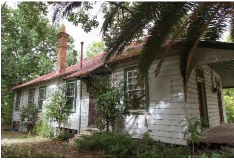
Figure 7: East elevation of former Police Station with original main entry.
