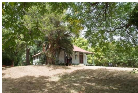
Figure 5: North elevation of former Police Station, viewed from Punt Road.
