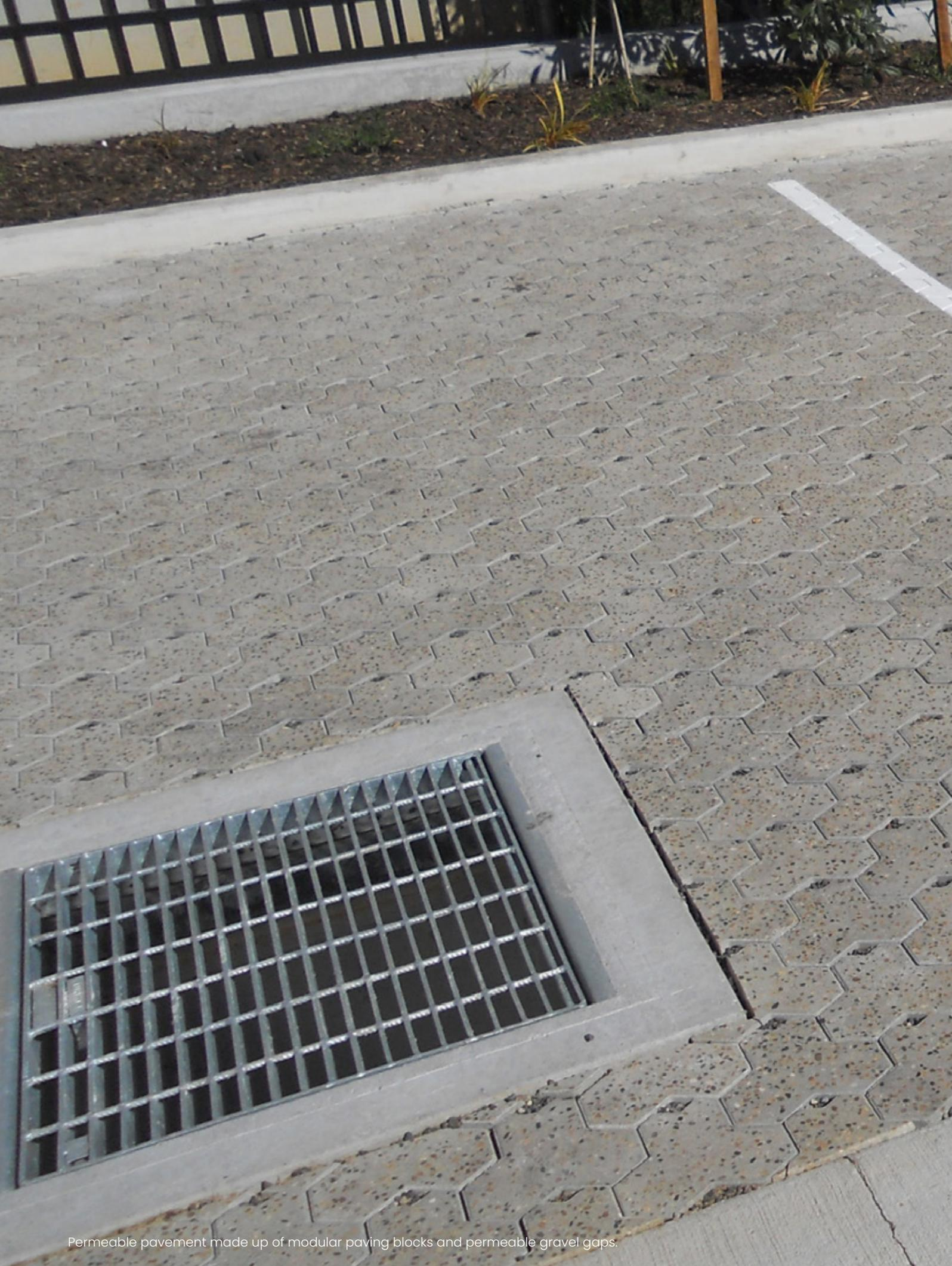
Permeable pavement made up of modular paving blocks and permeable gravel gaps.
