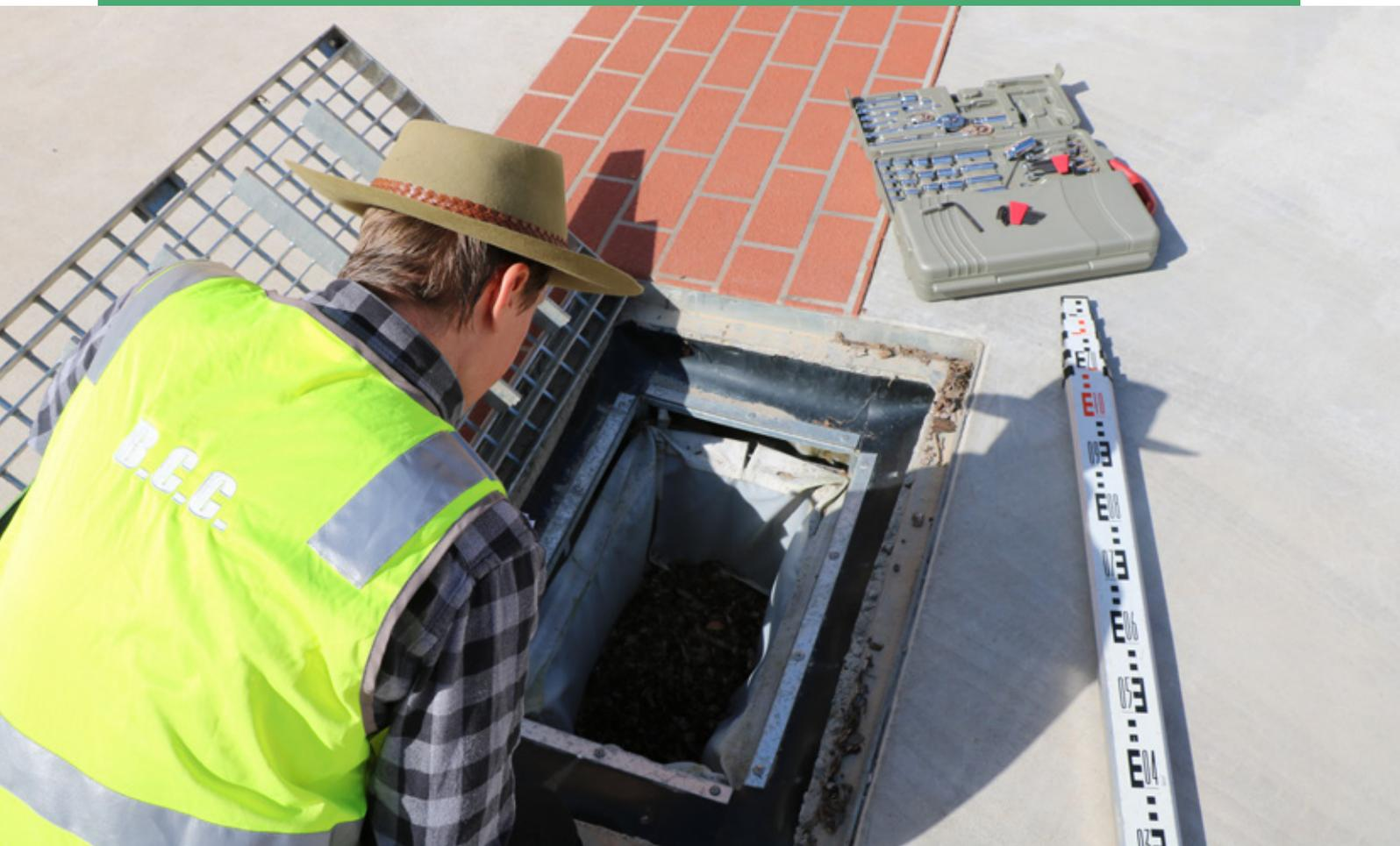
These devices are fitted into stormwater drainage pits to capture litter, debris and other pollutants from urban runoff. They are often used as the primary treatment of stormwater before it enters a secondary or tertiary treatment system.
