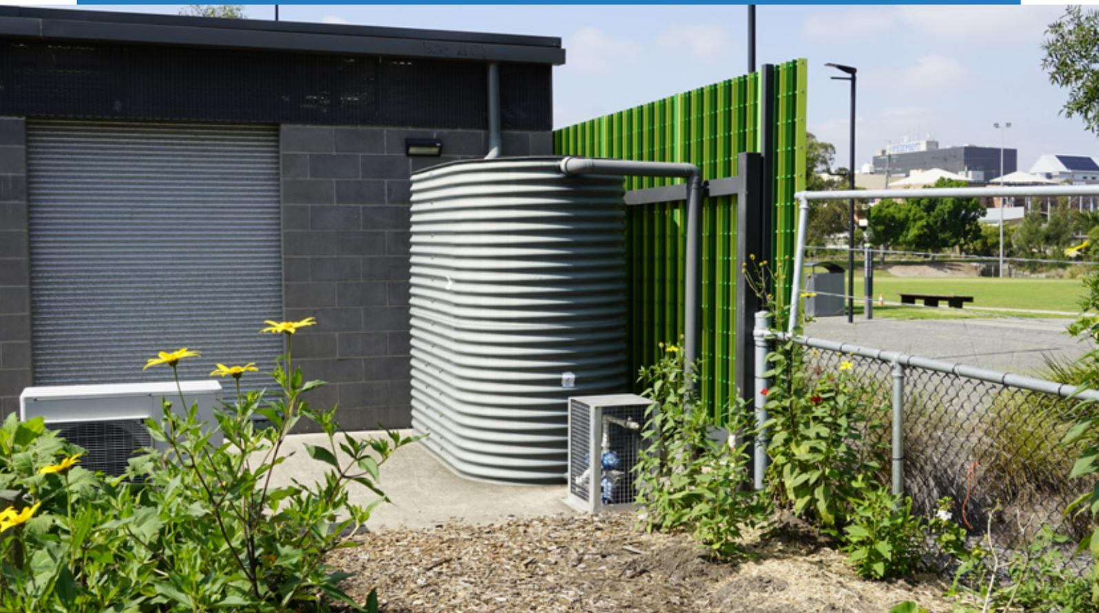
A rainwater tank captures and stores roof water for reuse on-site. It may also play a part in local flood control.
