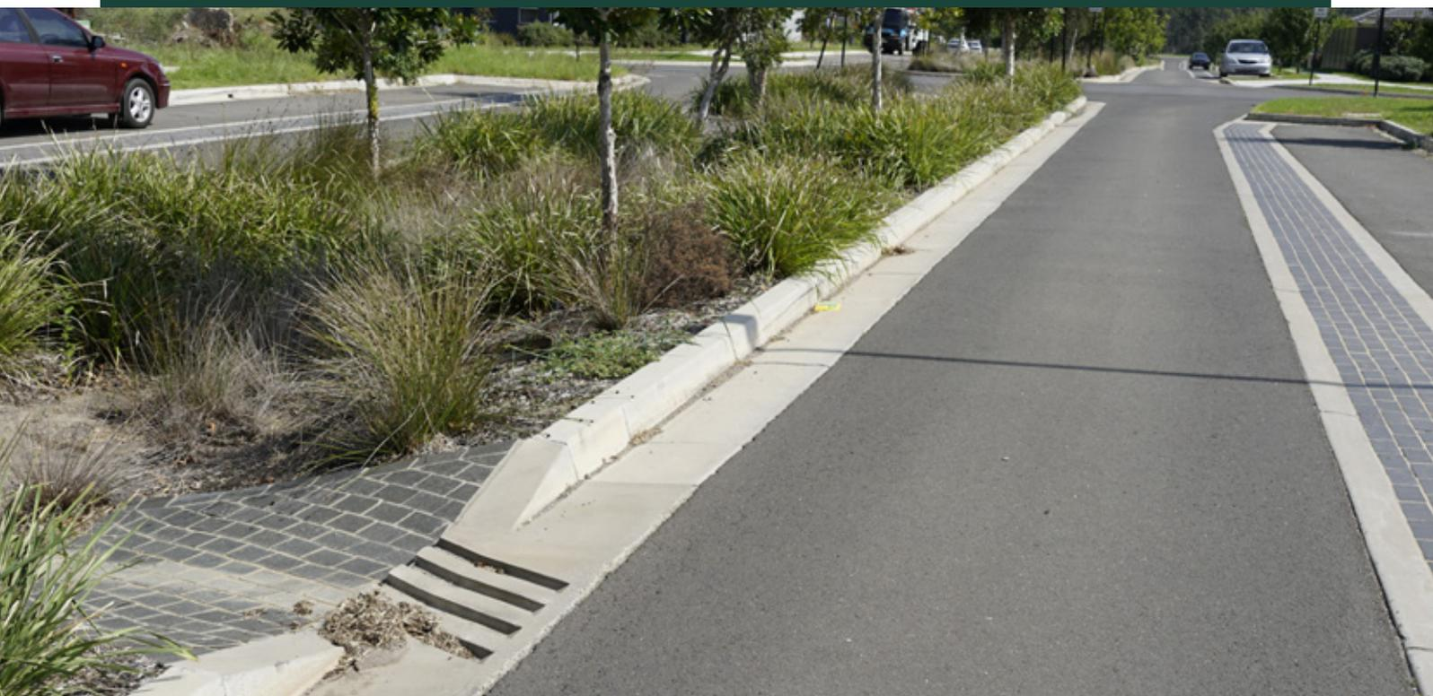
Vegetated buffer strips and swales are simple stormwater transfer systems that treat runoff through filtration and sediment capture. Buffer strips are vegetated surfaces (usually grassed) that allow runoff to flow towards a downstream outlet. Swales generally form a sloped vegetated channel that conveys stormwater along a long path. In both systems, water is slowed and filtered as it flows through the vegetation, capturing large sediments and absorbing stormwater runoff.
