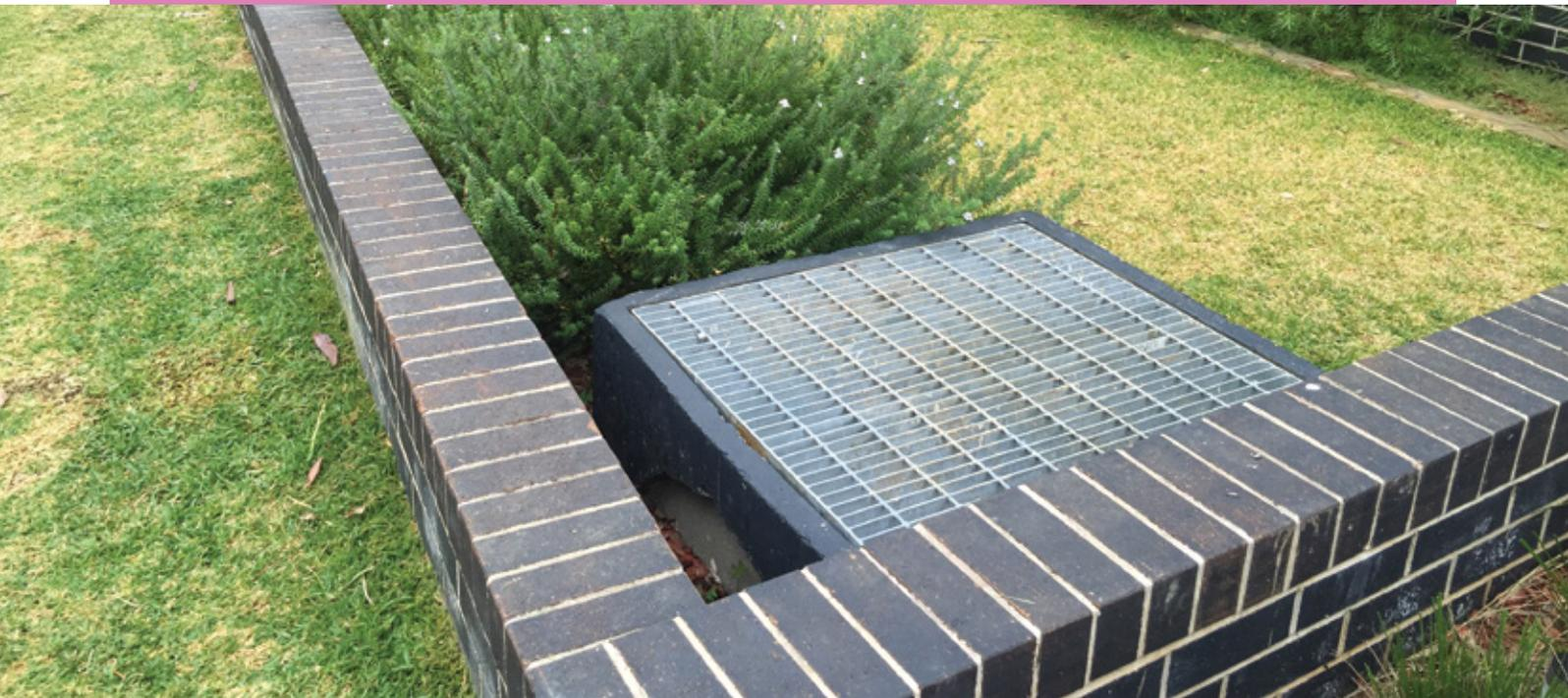
On-site stormwater detention (OSD) is the temporary storage and controlled release of stormwater generated on-site. OSD temporarily stores and slows down the rate of stormwater runoff from a property so that it does not worsen flooding downstream, whereas a rainwater tank stores rainwater.
