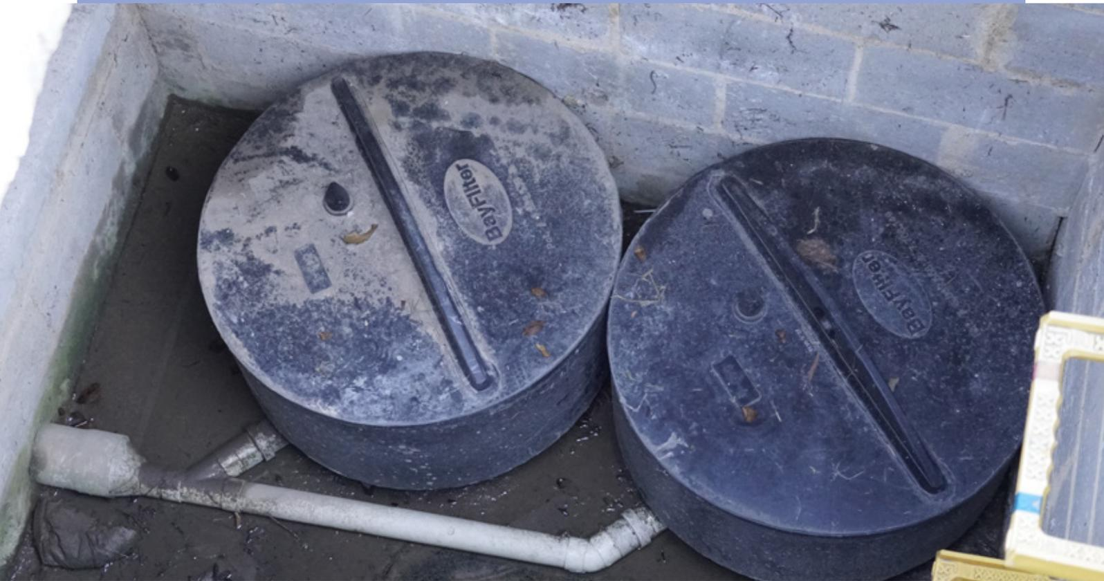
Filter cartridges include sand filters and proprietary products that operate in a similar way to GPTs, but are designed to filter finer pollutants, such as fine solids, soluble heavy metals, oils and nutrients.
