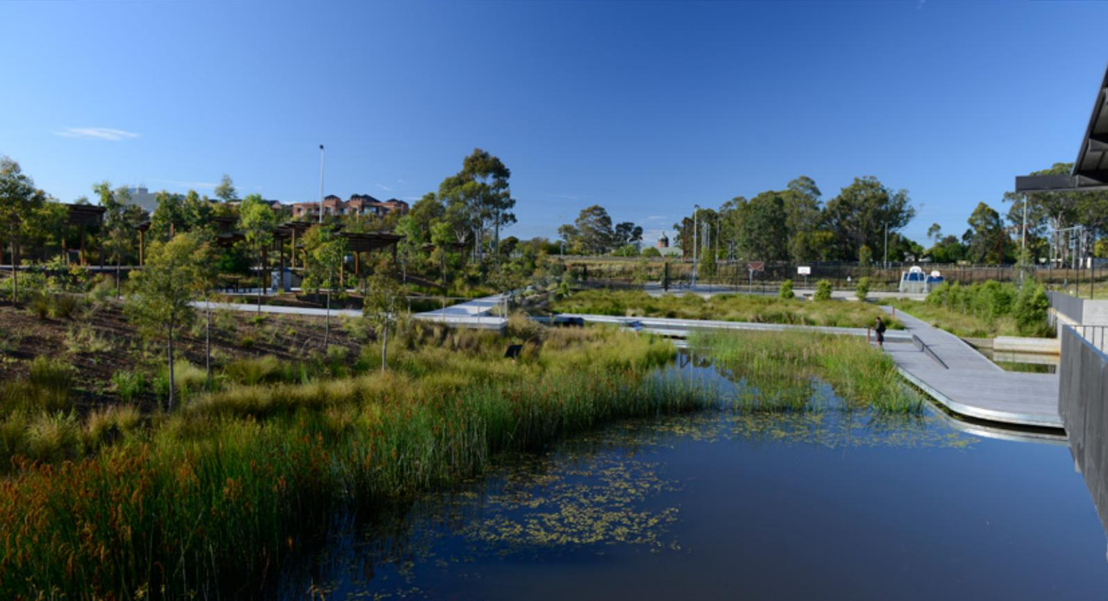
A wetland is a vegetated wet basin (or series of wet basins) that filter and treat stormwater before it enters our waterways. The plants in a wetland capture fine particles and absorb nutrients from the stormwater; they slow and filter the water allowing sediment to settle. Wetlands commonly have a gross pollutant and sediment trap upstream of them to capture coarse material before it enters the main part of the wetland (the macrophyte zone).
