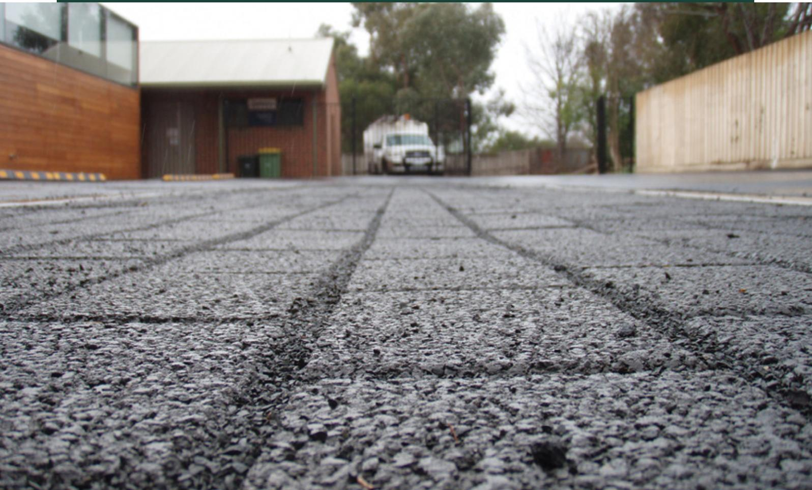
Permeable paving allows water to infiltrate through the paving, reducing the volume of runoff from hard surfaces such as roads, car parks and footpaths. This reduces local flooding and surface ponding, and promotes infiltration.
