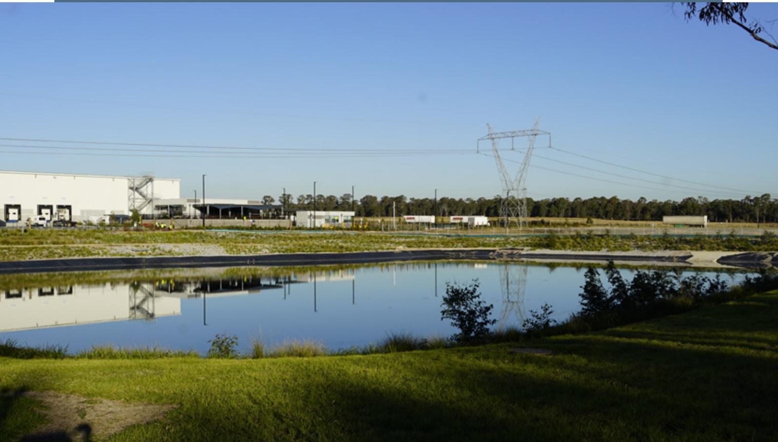
Temporary sediment basins are installed during the construction stage of a development to help manage stormwater impacts during construction. These open water bodies treat stormwater by allowing coarse particles and suspended sediments to settle.
