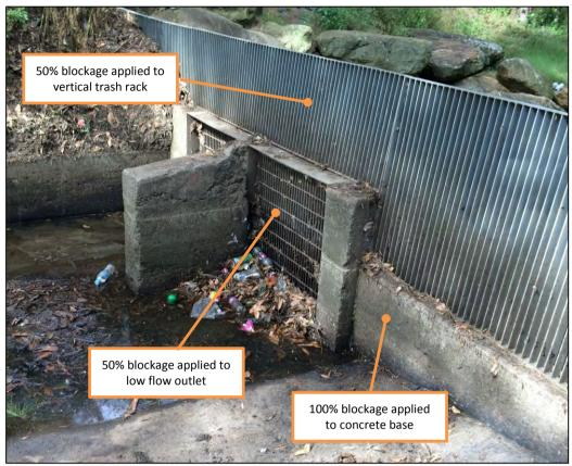
Plate 2 View showing downstream trash rack
