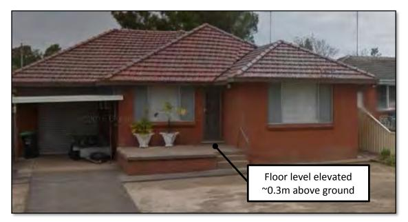
Plate 4 Example of a building on Stafford Street showing the building floor level elevated by about 0.3 metres above the adjoining ground surface
