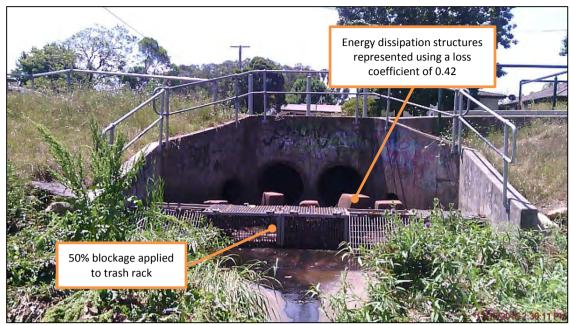
Plate 6 View looking towards Herbert Street showing energy dissipation structures and trash rack
