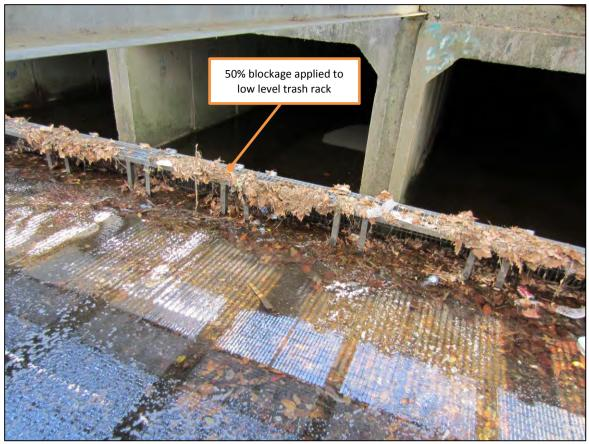
Plate 4 Low level trash rack located within inlet pit
