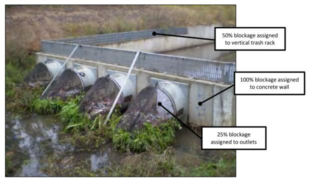
Plate 9 Irwin Street GPT showing concrete wall, trash rack and outlet pipes with debris nets
