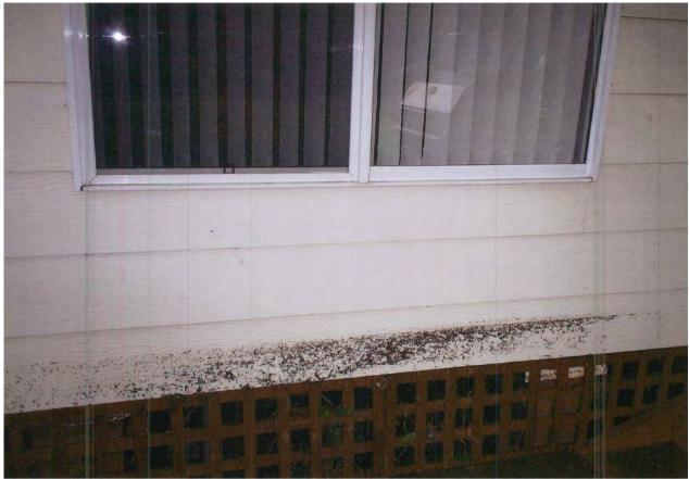
Flooding under floor at 4 Shaw Street (estimated to be 50cm depth)
