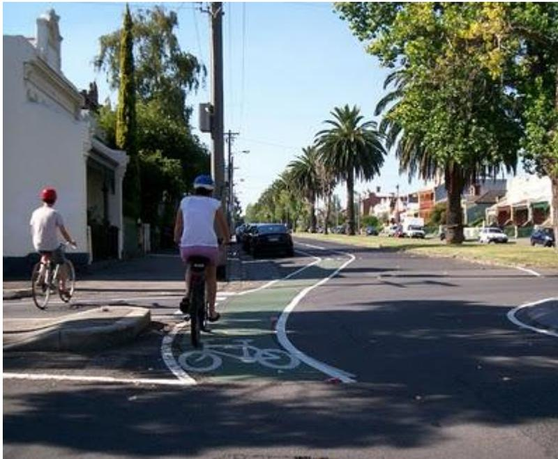
Note - Use of colour to delineate a cycle lane through a roundabout in Canning St. - Melbourne
