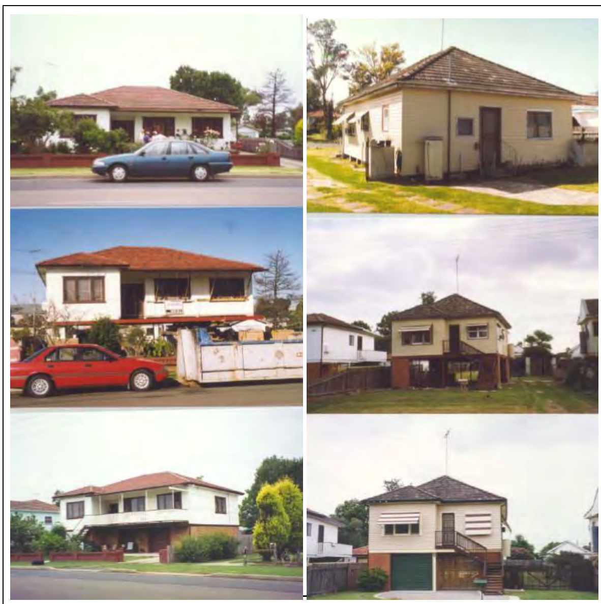
Plate 58 Examples of houses before (top image), during (middle image) and after (bottom image) house raising (photos courtesy of Fairfield City Council)
