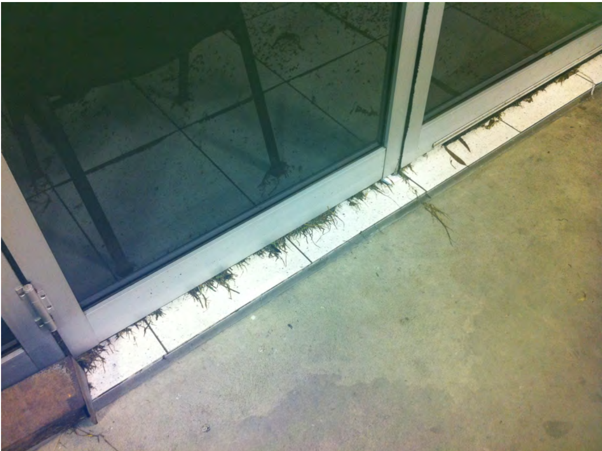
Above floor inundation at Morley Ave, Kingswood
