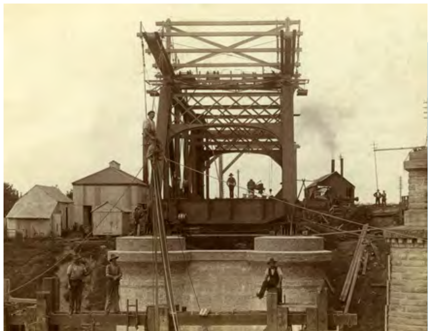
Penrith rail bridge under construction in the early 1900s
