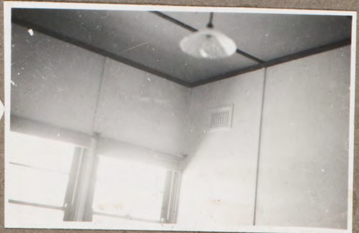
Note the use of large slabs saving timber and above all (Are you listening, Mr. Tojo?) saving manpower.
