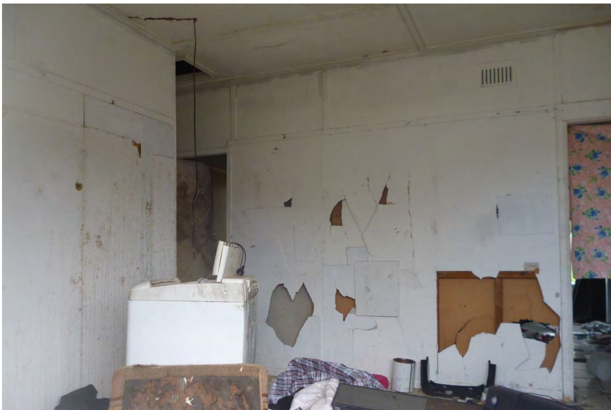
Figure 13: Internal view of living area in Duration Cottage located at 45 Carinya Avenue.
