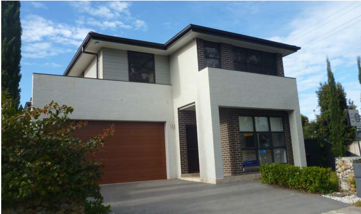
Figure 8: One of the contemporary houses, located at 9 Kalang Avenue, constructed post demolition of Duration Cottage, view looking southeast.
