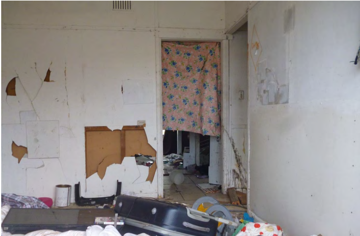
Figure 14: Internal view of living area in Duration Cottage located at 45 Carinya Avenue.
