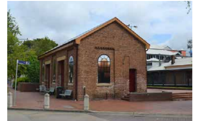
Fig. 19: Heritage goods shed outside the train station
