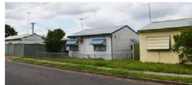
Fig. 23: St Marys Duration Cottages
