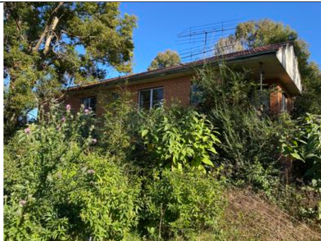
Photograph 15: Rear of house. View to west.
