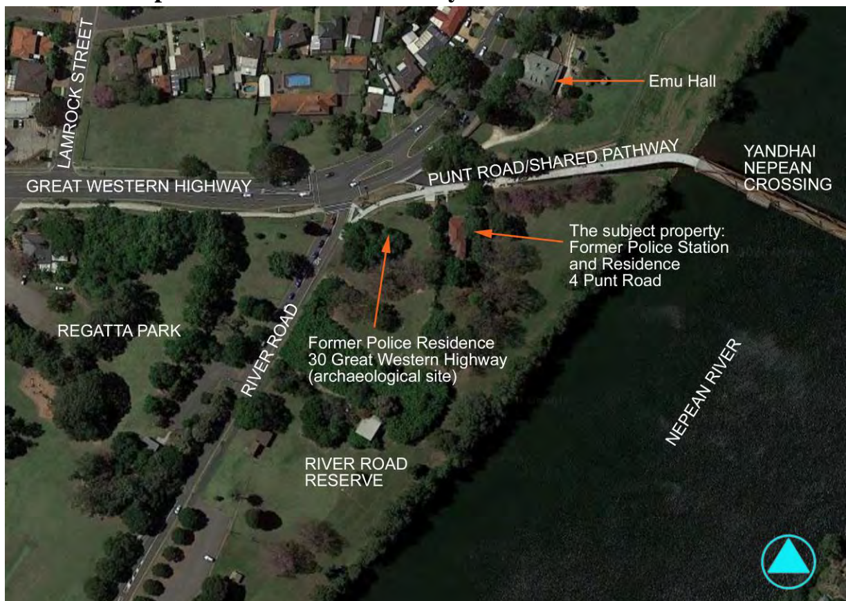
Figure 3. 1: Aerial view of place showing the key features. Source: GoogleMaps, 2020
