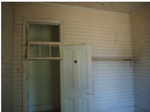
Figure 3. 67: S5 (bedroom) with door and broken fanlight.
