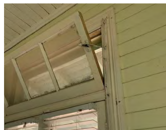
Figure 3. 85: Fanlight above door to S1.
