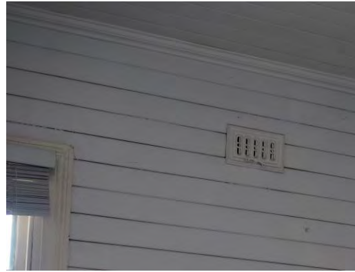
Figure 3. 87: Typical pressed metal air vent.
