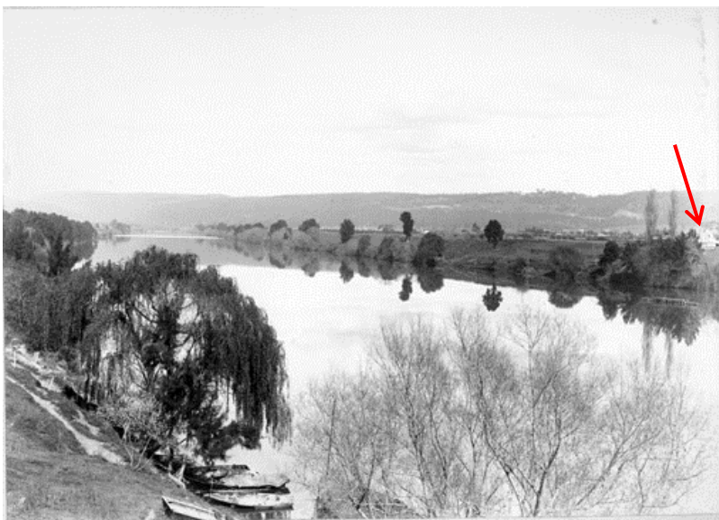
Figure 2. 25: 1890s photograph of the Nepean River. The Punt House is seen far right of frame (indicated with an arrow). Source: Penrith City Council, 1662
