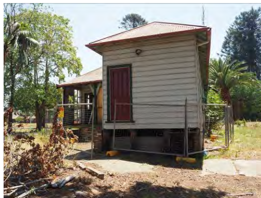
Figure 3. 44: South (rear) elevation of east wing extension.
