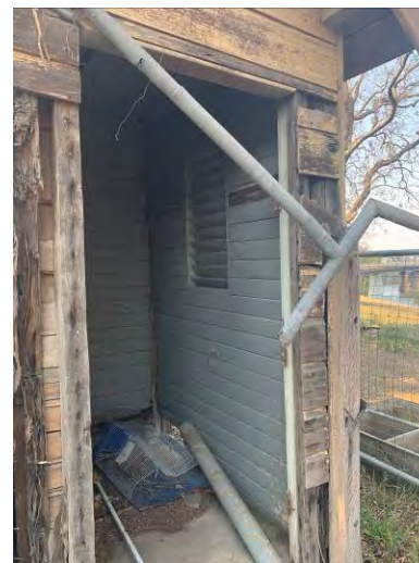
Figure 3.97: Interior view of south space.
