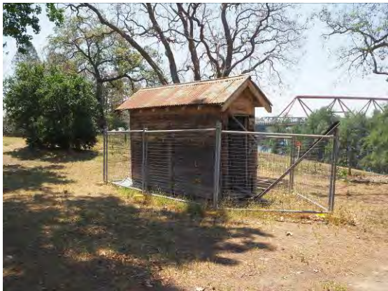
Figure 3.91: West and south elevations.
