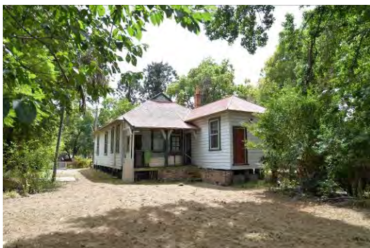
Figure 3. 45: South (rear) elevation.
