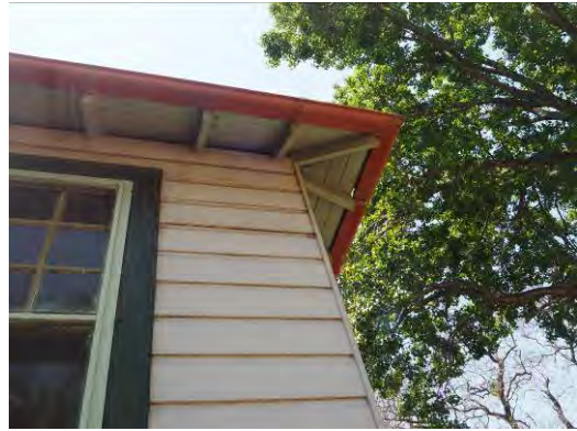
Figure 3. 52: Detail of external weatherboards and timber panelled soffits and exposed eaves rafters.
