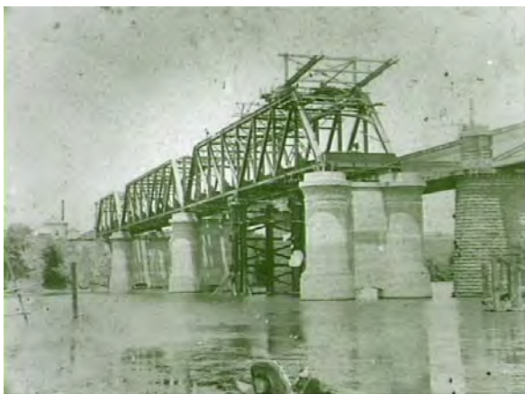
Figure 2. 22: 1906 photograph of the Victoria Bridge and the rail bridging under construction. Source: Penrith City Council, 608
