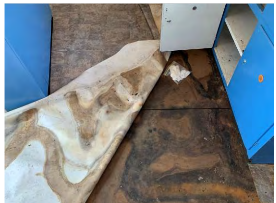
Figure 3. 78: Vinyl floor covering in S9 (kitchen).
