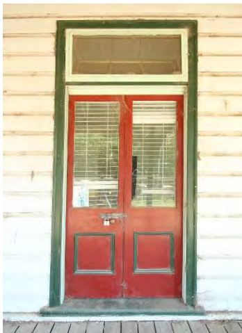
Figure 3. 55: Door to northern elevation.
