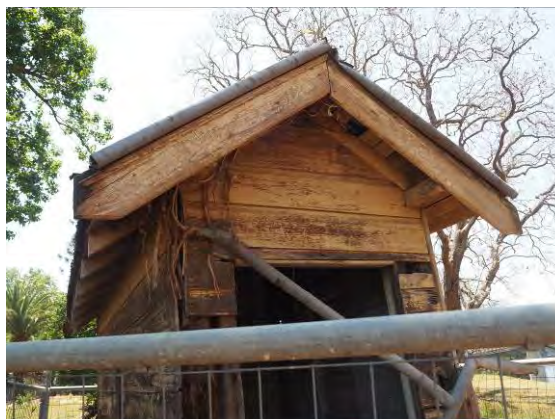
Figure 3.94: Detail of barge board, timber panelling to soffits and exposed eaves rafters.
