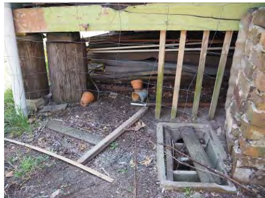
Figure 3. 54: View of roof sheeting and other building elements stored under the building.
