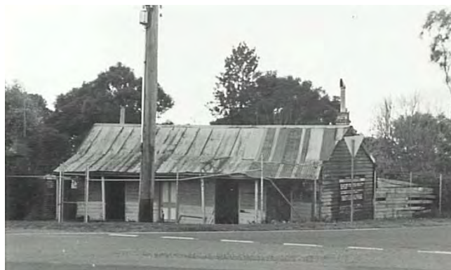
Figure 2. 29: Undated (1980s) photograph of the former cottage at 30 Great Western Highway. Source: Penrith City Council
