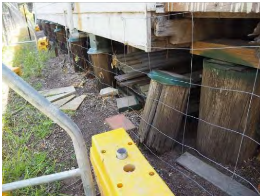
Figure 3. 53: Timber log piles with ant caps.
