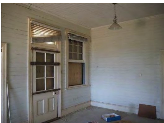
Figure 3. 71: S6 (living room) with door and window leading to south (rear) verandah.
