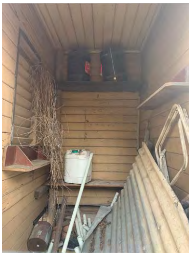
Figure 3.95: Interior view of north space.
