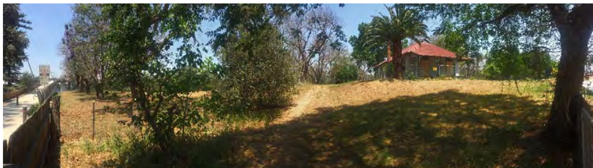
Figure 3. 27: View to the former police residence from Punt Road showing the pronounced bench on which the house is sited and an earlier access track from Punt Road. The date palm next to the house is an appropriate choice for the 1908 building.
