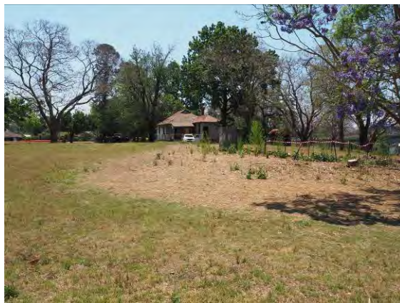
Figure 3. 11: Broad view of the cottage in its setting, looking northeast.
