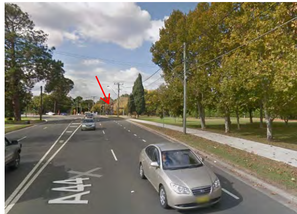
Figure 3. 18: View V4 from Great Western Highway looking east along road to west elevation of the residence amongst trees. The building is indicated with an arrow. Source: GoogleMaps/Streetview
