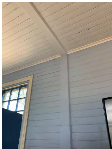
Figure 3. 80: S9 (kitchen) with evidence of location of former partition in ceiling and west wall.
