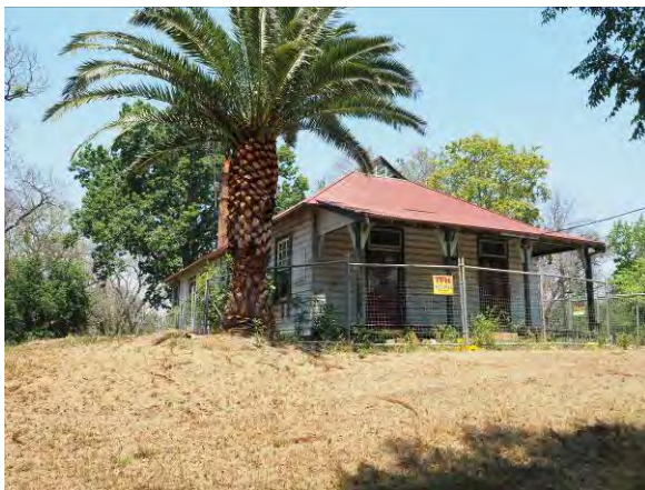
Figure 3. 8: The street frontage of the former Police Residence property in its landscaped setting.
