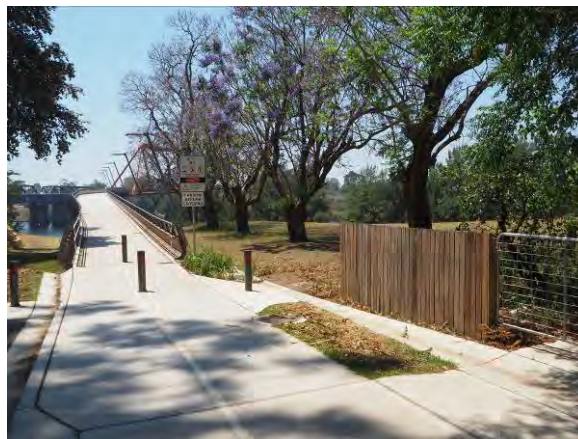
Figure 3. 3: view looking east along shared pathway to the pedestrian bridge crossing over the Nepean River.
