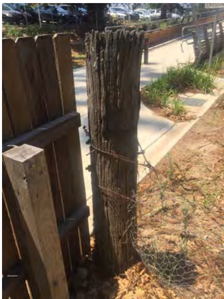
Figure 3. 32: A remnant timber post at Punt Road that forms the start of the earlier lot fence along the eastern site boundary. Note the strained wire and netting and the check for the missing timber straining brace.
