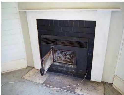
Figure 3. 70: S6 (living room) fire place with later addition surround and fire box and original concrete hearth stone.
