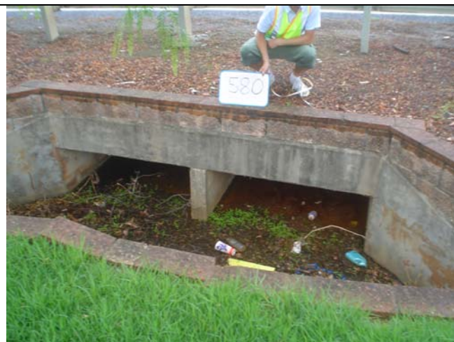
CLT ID No 580: 282532.62, 6258589.85 (Coordinates - MGA 94, Zone 56) Downstream end - dimensions: 2 x 1.6m (W) x 0.7m (H)
