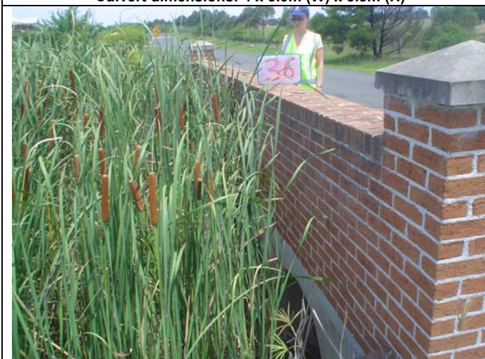
CLT ID No 36: Bowood Way, Mt. Vernon Upstream side. Culvert dimensions: 4 x 1.1m (diameter)
