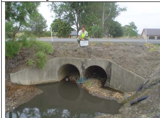
CLT ID No 579: 286952.01, 6258171.34 (Coordinates - MGA 94, Zone 56) Culvert dimensions: 2 x 1.1m diameter
