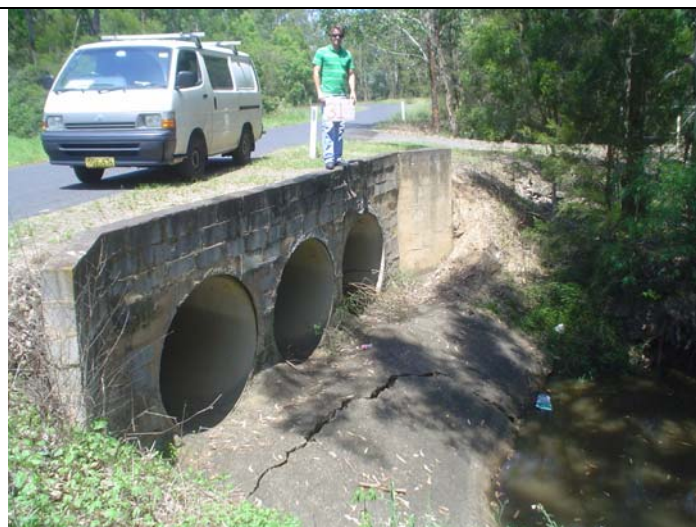
CLT ID No 31: Bowman Rd, Londonderry Culvert dimensions : 3 X 1.6m diameter culverts
