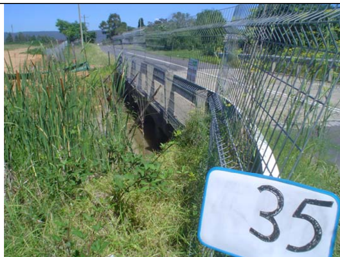
CLT ID No 35: Nepean Street, Mt. Pleasant Culvert dimensions: 4 x 2.5m (W) x ~1m (H)
