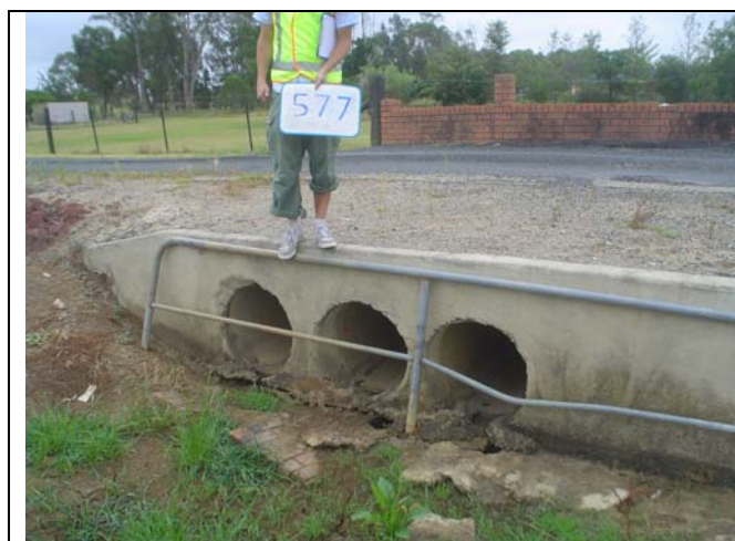
CLT ID No 577: 286857.81, 6258082.76 (Coordinates - MGA 94, Zone 56) Bridge dimensions: 3 x 0.6m Diameter
