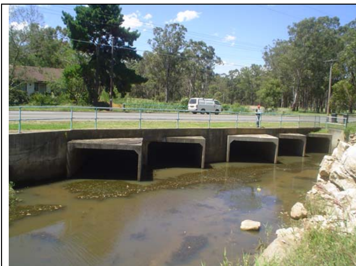
CLT ID No 30: Victoria Street, Kingswood Culvert dimensions: 5x3.2 (W) x2 (H)
