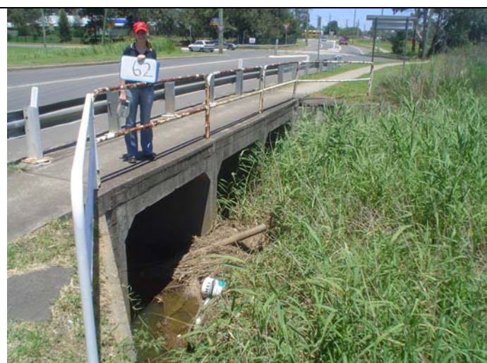
CLT ID No 62 Werrington Road, Werrington Culvert dimensions: 3 x 2m(W) x 1.8m(H)
