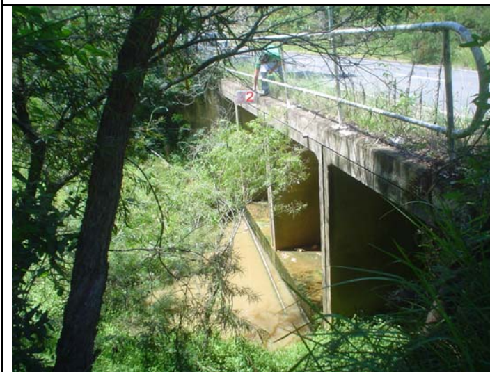
CLT ID No 32: Carrington Road, Londonderry Culvert dimensions: 4 x 3.0m (W) x 3.8m (H)
