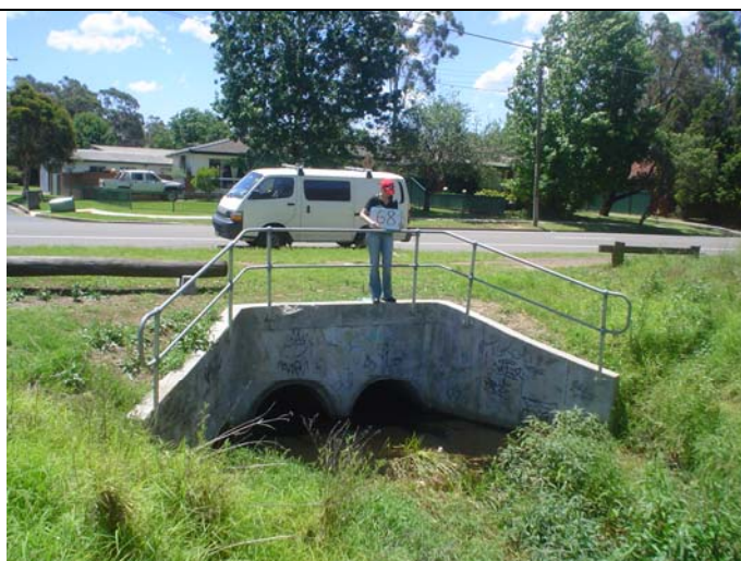
CLT ID No 68: Shaw Park, Cambridge Park 2 x 0.9m diameter pies and 1 x 0.6m diameter pipe
