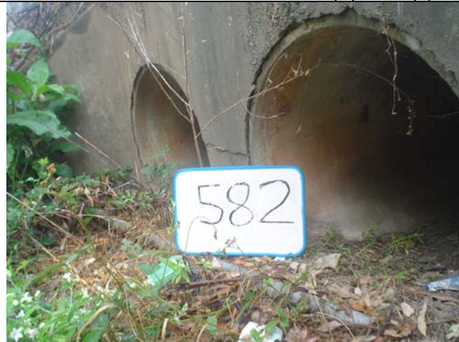
CLT ID No 582: 282429.81, 6259154.47 (Coordinates - MGA 94, Zone 56) Dimensions: 2 x 0.7m Diameter
