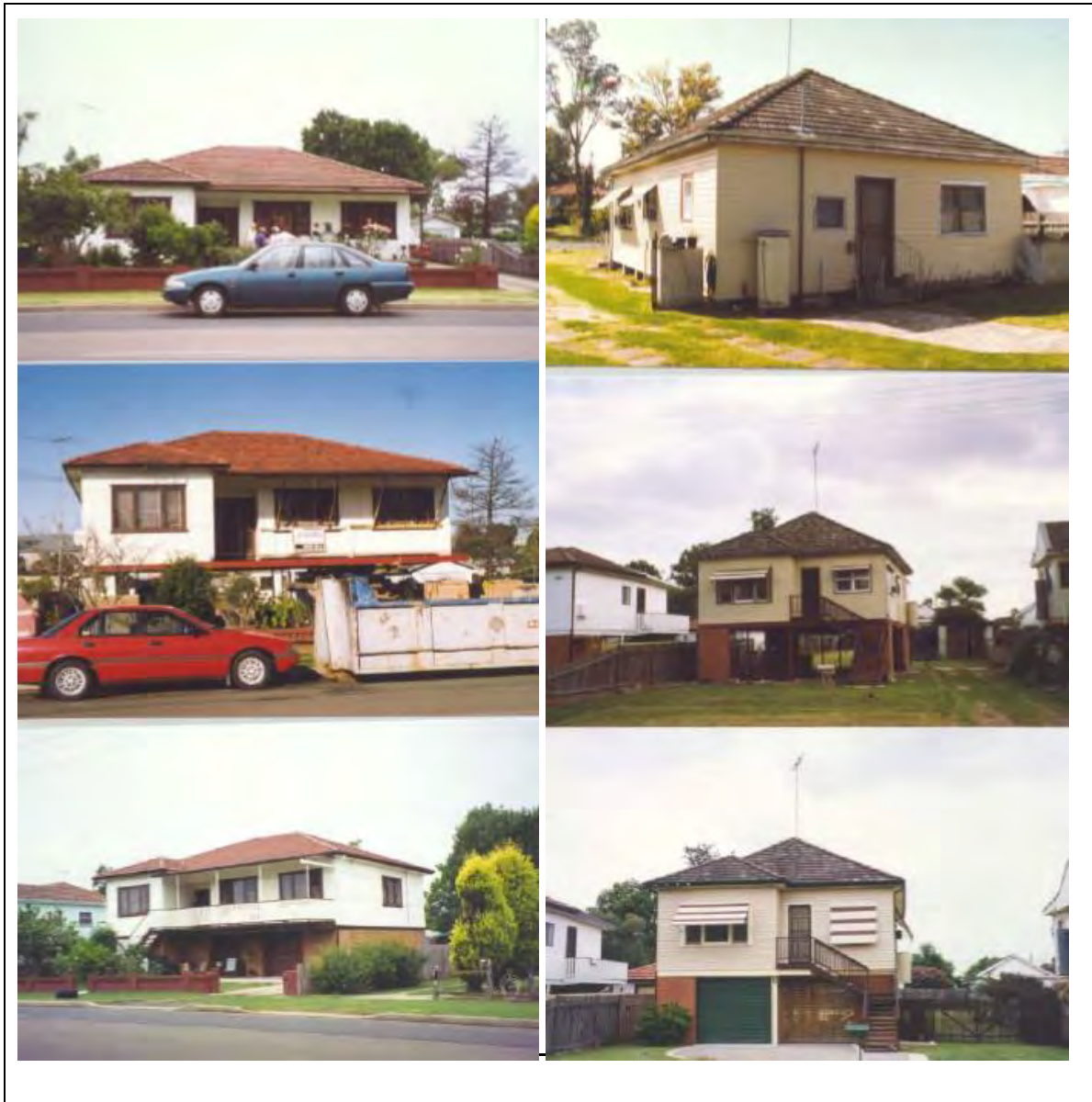
Plate 42 Examples of houses before (top image), during (middle image) and after (bottom image) house raising (photos courtesy of Fairfield City Council)
