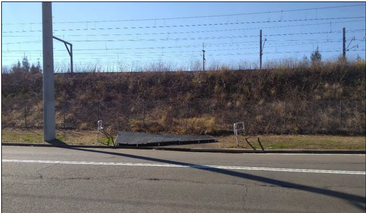
Plate 22 View looking north showing Hobart Street in foreground, stormwater inlet pit and elevated railway embankment
