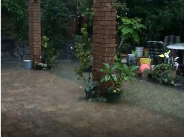
Plate C1.1 – (Photo taken at 19:00 hours) Floodwater ponding in rear of property that is located on Soling Crescent, Cranebrook.
