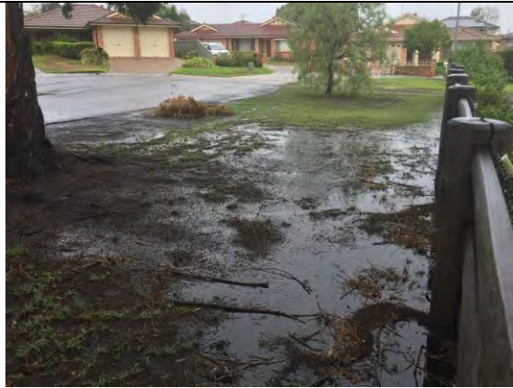
Plate C4.1 – Floodwater ponding between road and front of properties that are located on the western side of Linden Crescent, Cranebrook.
