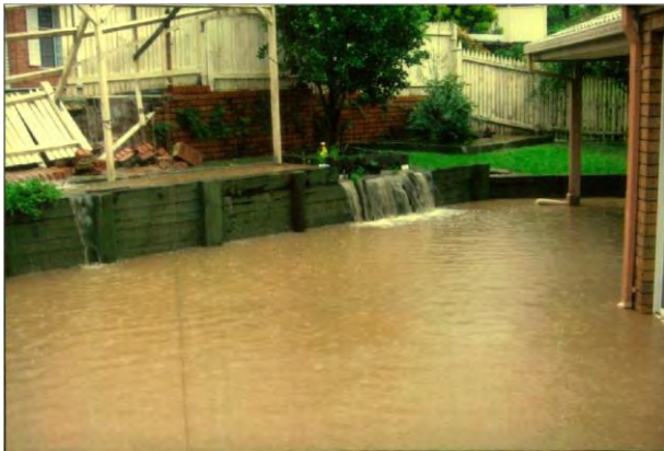
Plate C6.3 – Flooding at rear of property that is located on Waterfall Crescent, Cranebrook.
