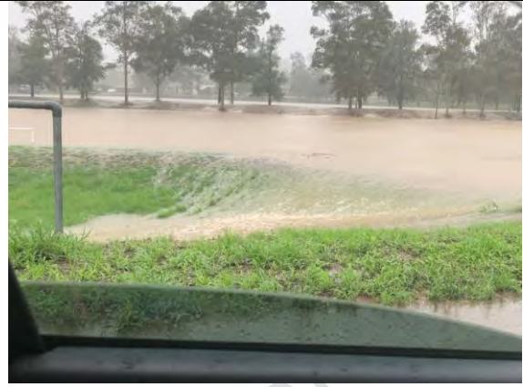
Plate C5.2 – (Photo taken at 15:00 hours) Floodwater surcharging the spillway of the Borrowdale Road Basin No. 2.
