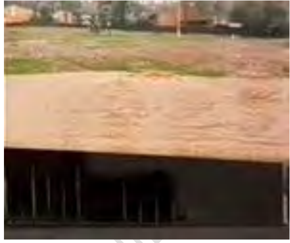
Plate C6.2 – Location not specified.
