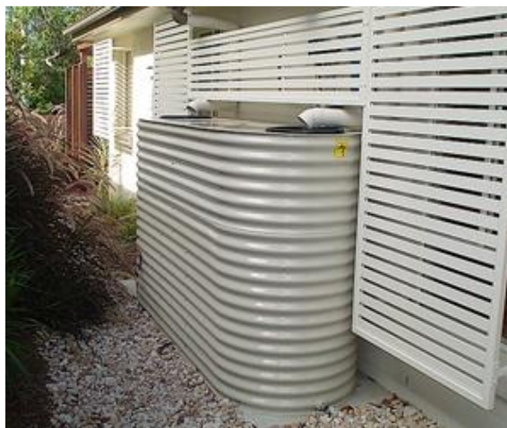
Figure 4.1: Rainwater tank (source: www.savewater.com.au )
