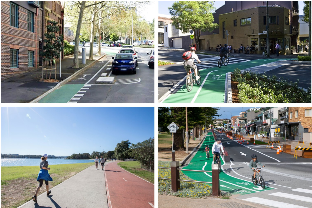
Top left: Uni-directional cycleway, Campbell Street, Surry Hills (City of Sydney); Top right: crossing of bi-directional cycleway, Bourke Street, Surry Hills (City of Sydney); Bottom left: separated cycle path and pedestrian path, Bay Run, Rozelle (Inner West Council); Bottom right: Semi-permanent bi-directional cycleway, The Strand, Dee Why (Northern Beaches Council)
