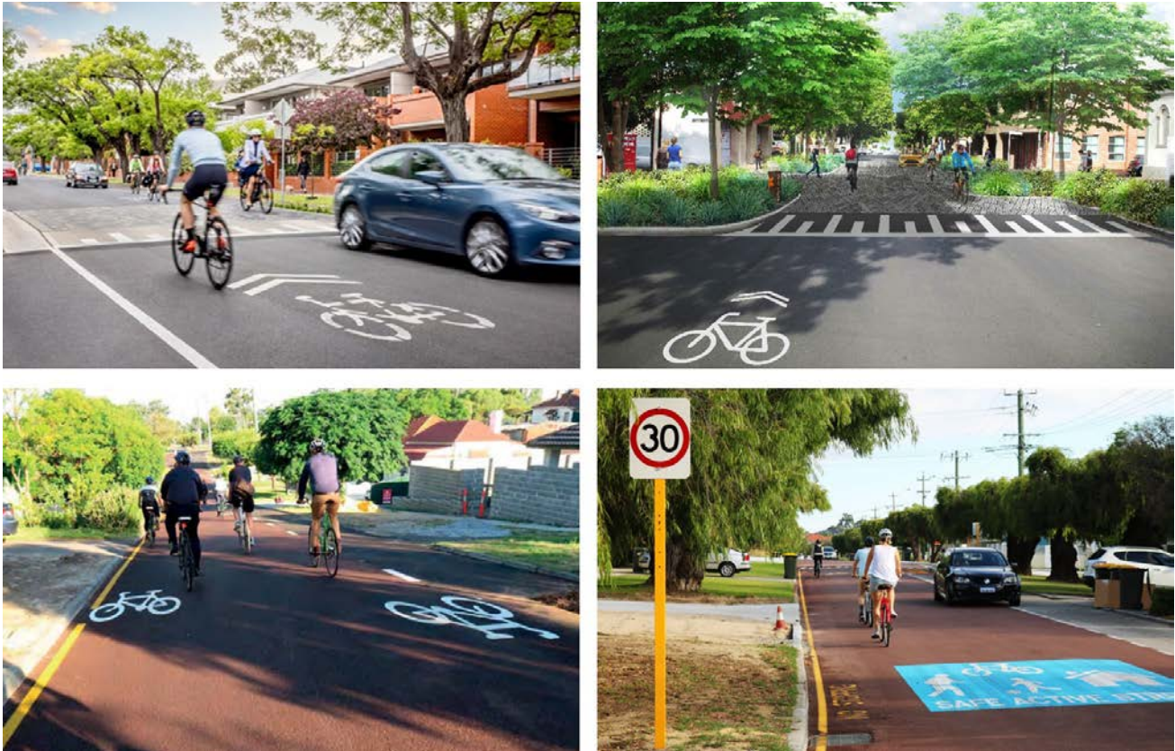
Top row: Bicycle Quietway / Boulevard with traffic calming and contrasting pavement surface – Beulah Road, Norwood (Adelaide SA) Bottom left: Bike Quietway using red asphalt – May Street, Bayswater (Perth WA), Bottom right: Reduced speed limit and red asphalt – Shakespeare Street, Mount Hawthorn (Perth WA)
