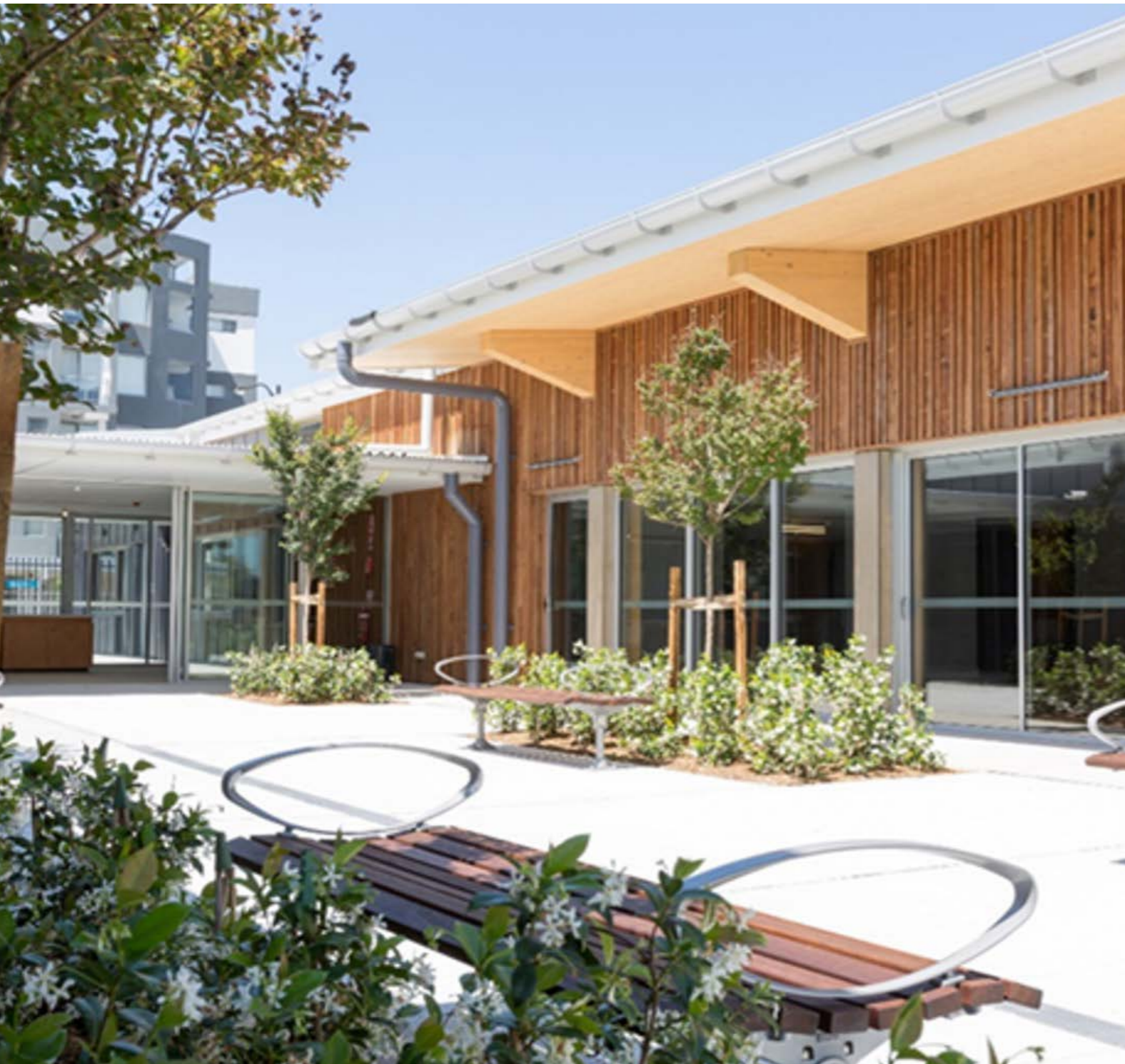
Jordan Springs Community Hub, source: Penrith City Council.
