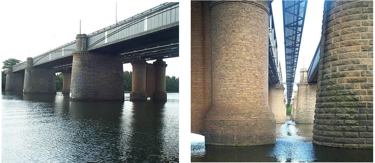
Figure 9 - Photographs of Victoria Bridge piers
