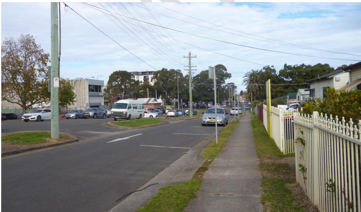
Figure 4: Open car park and commercial development along Carinya Avenue opposite the Duration Cottages precinct, view looking southeast. The car park was created by demolition of a row of Duration Cottages that were built at the eastern side of Carinya Avenue.
