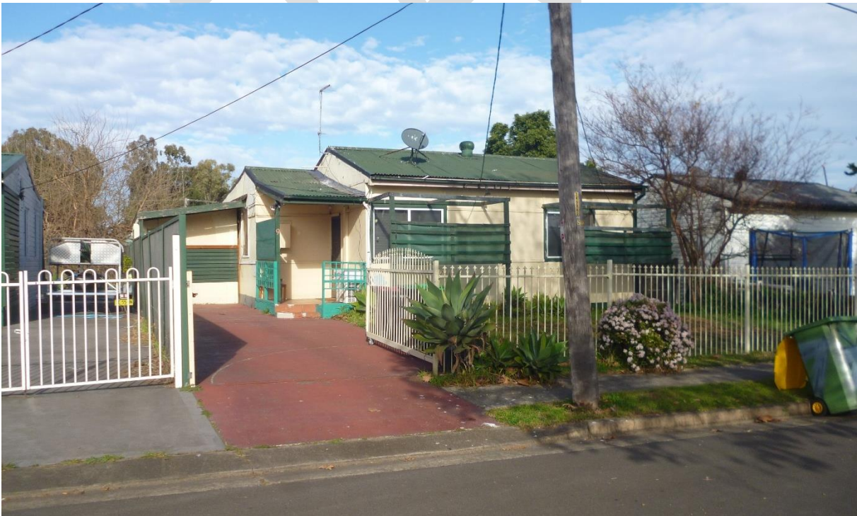
Figure 7: View of Cottage located at 9 Camira Street, view looking southwest.
