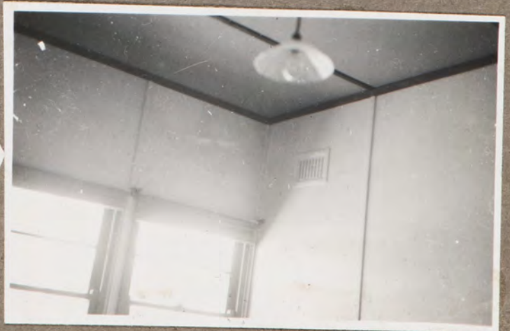
Note the use of large slabs saving timber and above all (Are you listening, Mr. Tojo?) saving manpower.
