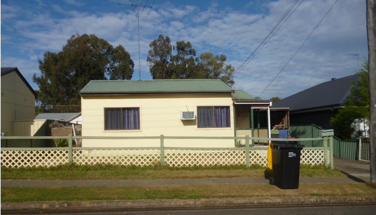
Figure 6: View of cottage located at 9 Nariel Street, view looking south.
