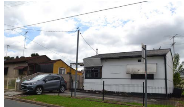
Fig. 68: Small footprint 'Duration Cottage' on a narrow lot to the west of Queen Street
