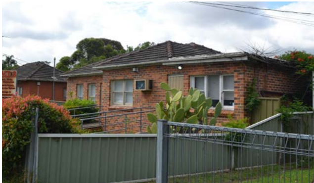
Fig. 65: Single storey detached dwelling - the most common typology of housing in the Study Area
