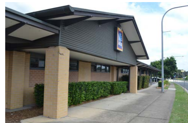
Fig. 79: Facade with awning but no active frontage
