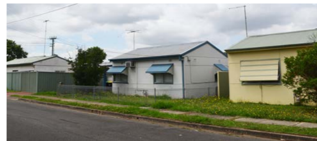
Fig. 23: St Marys Duration Cottages
