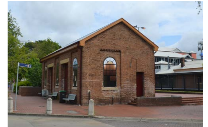
Fig. 19: Heritage goods shed outside the train station
