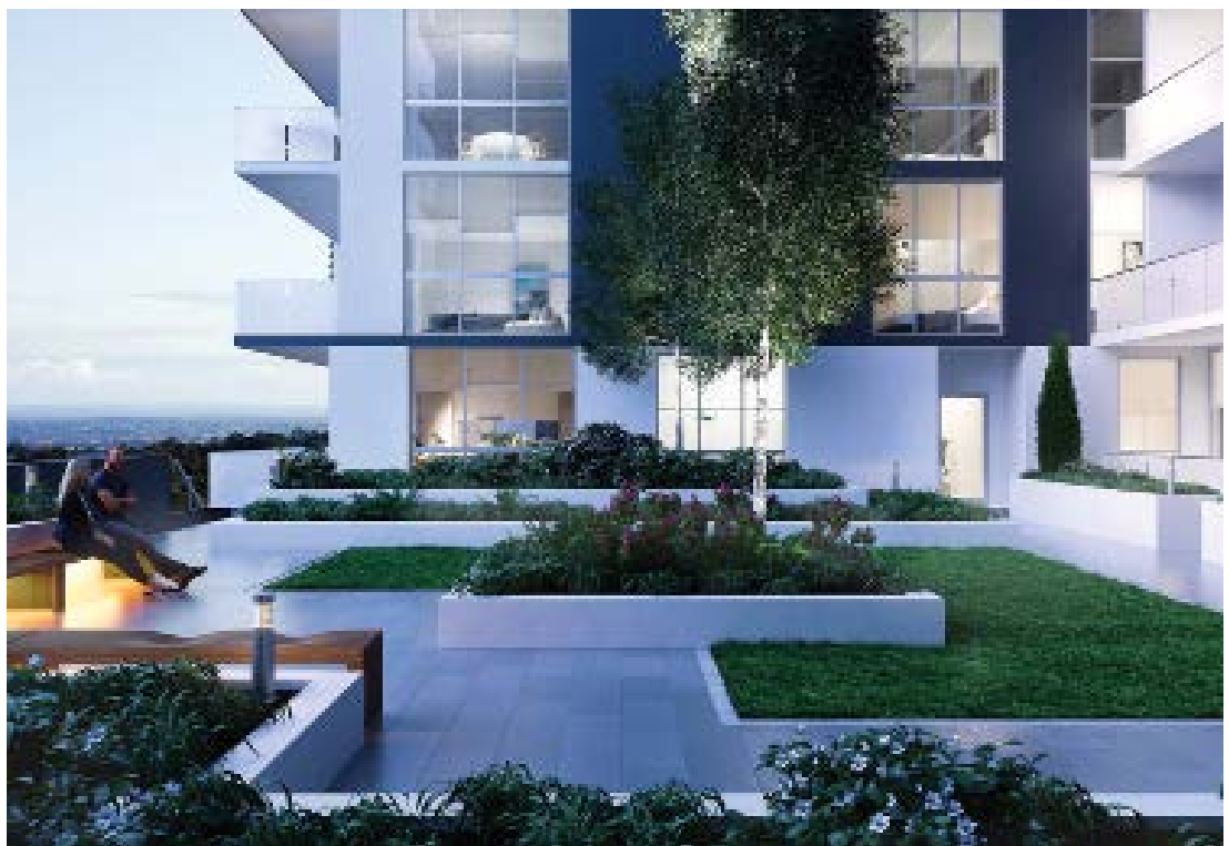
Figure 39: Harts Landing development in Thornton, where half of all units are affordable units.
