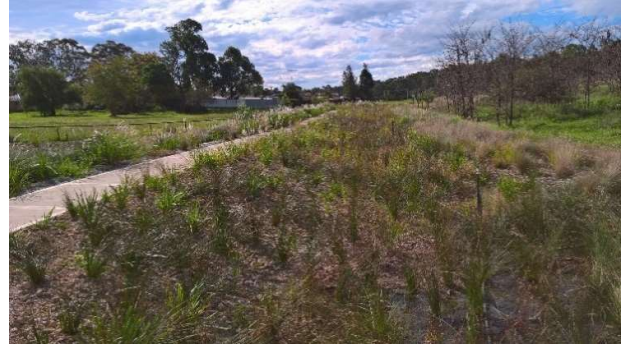
Figure 3: WSUD bioretention (Raingardens) basins and wetlands in Penrith LGA
