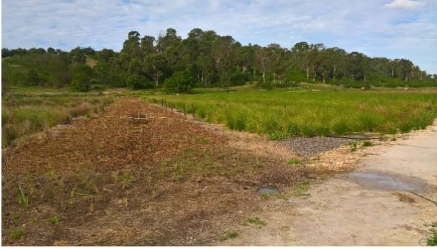
Figure 3: WSUD bioretention (Raingardens) basins and wetlands in Penrith LGA
